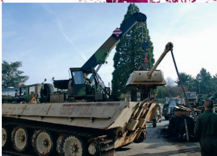
➤ The heavy operations, like the turret removal, remain in the hands of the Armor school professional mechanics.
